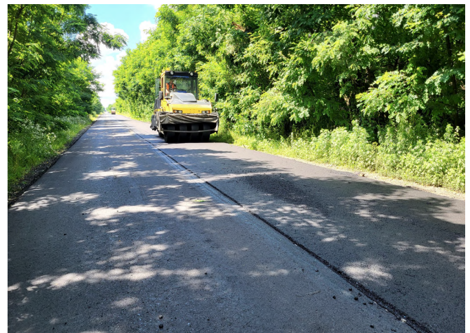
A road maintenance between Vyshhorod (the Kyiv region) and Chernihiv
